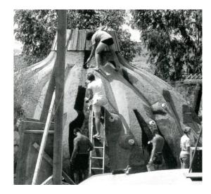
Left to Right: Figure 33 - Completed concrete casting Figure 34 - Removal of silt when concrete has set
